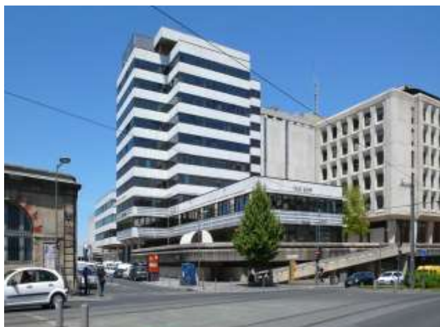
Photo Sauvegarder Mériadeck
