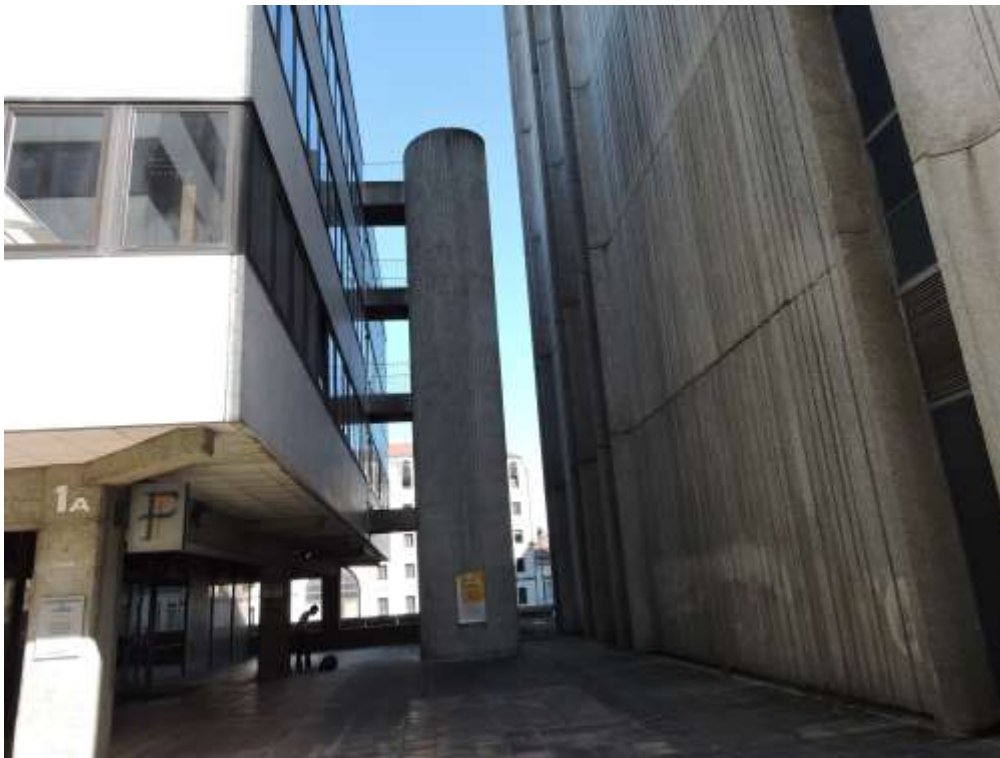
Photo Sauvegarder Mériadeck
