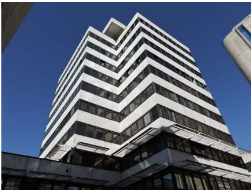
Photo Sauvegarder Mériadeck
