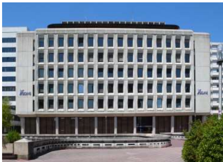
Photo Sauvegarder Mériadeck
