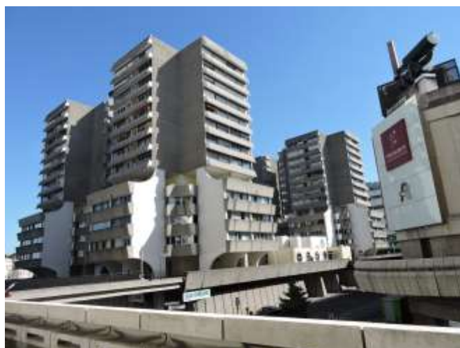
Photo Sauvegarder Mériadeck
