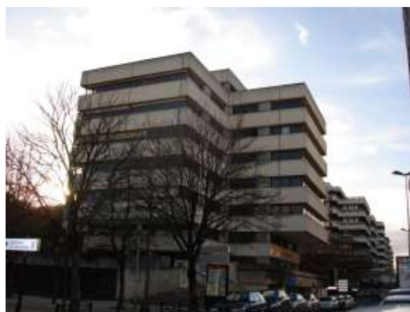
Photo Sauvegarder Mériadeck
