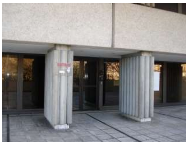
Photo Sauvegarder Mériadeck
