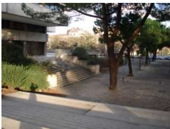
Photo Sauvegarder Mériadeck
