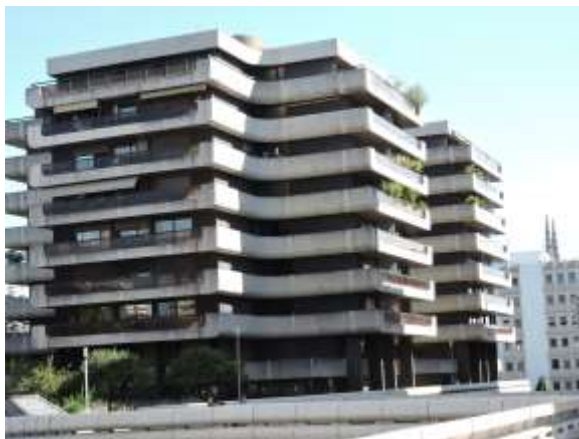
Photo Sauvegarder Mériadeck
