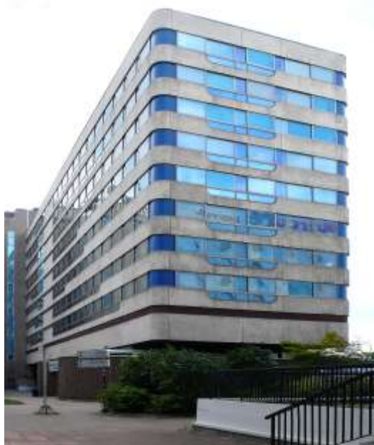
Photo Sauvegarder Mériadeck
