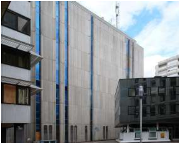
Photo Sauvegarder Mériadeck
