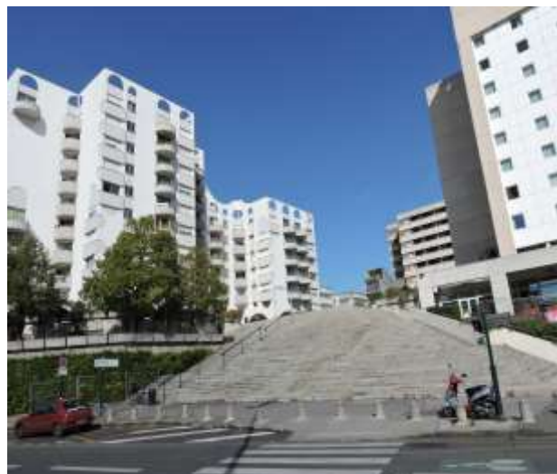
Photo Sauvegarder Mériadeck
