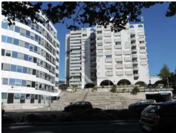
Photo Sauvegarder Mériadeck
