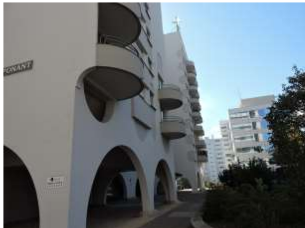
Photo Sauvegarder Mériadeck
